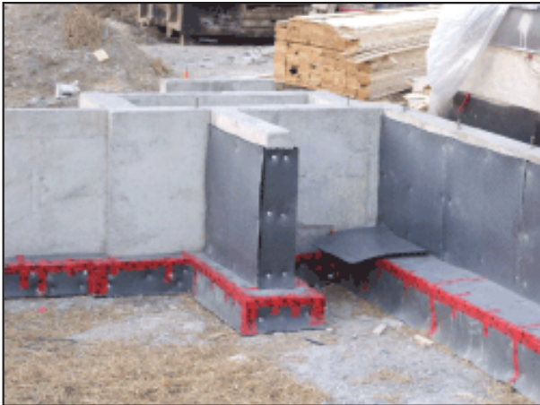
Building footings isolated from ground borne vibration using single layer Iso-Sep 25HD . Fastener heads to be covered with isolation pads.
