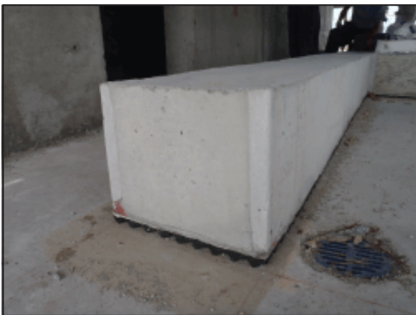
Properly isolated concrete pier for heavy equipment for example: chillers or cooling towers - Iso-Sep 25HD for lighter, and Iso-Sep 25F for heavier applications.
